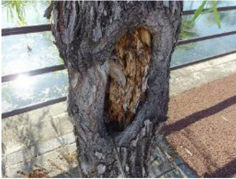
開口空洞・腐朽
